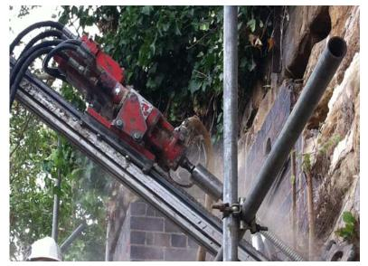
Piletec's Rig Operator said he was very impressed with the strength of the SEA hollow bar with larger diameter hole which improved flushing and grouting speeds. The adaptor worked very well and unlike others, the bar did not seize in the drive but remained loose allowing for easy removal and additional lengths to be added without delay. Thanks to SEA the project was on time and within budget.
